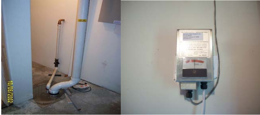
(Sump pit connection; system indicator & power converter)
